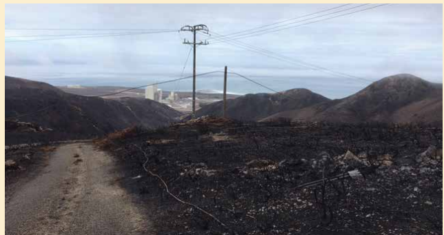
Concrete poles after fire broke at Vandenberg Air Force Base, California
